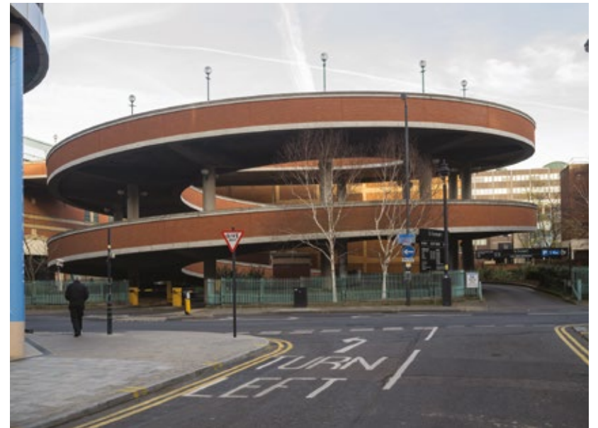
Multi-storey car park, Kymberley Road © Philipp Ebeling
