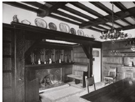
Inglenook Fireplace © H. Bedford Lemere
