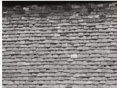
Hanging Tiles © Graham Horn
