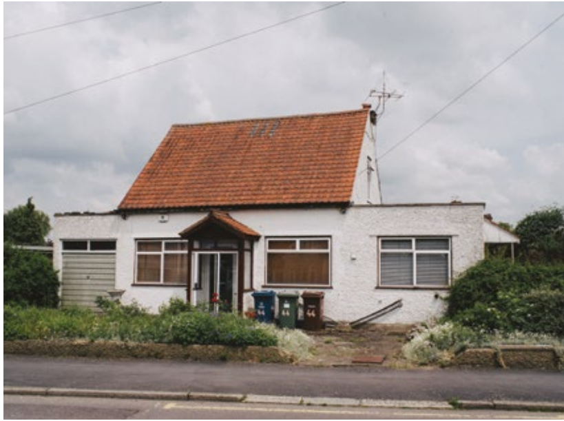
Extension, South Harrow © Philipp Ebeling
