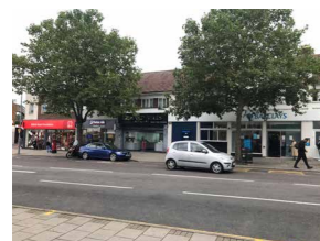
Chingford Mount Road Streetscape to the east
