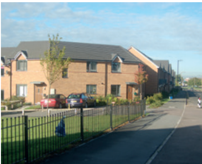
Surface treatment in front of dwellings and in car courts is often unclear as whether it is for pedestrians or cars.
