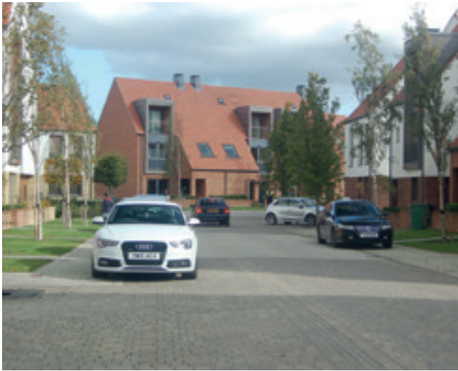
Access within the development is interrupted by cars parked on pavement surfaces.
